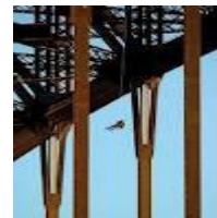
Rappelling the Sydney Harbour Bridge
