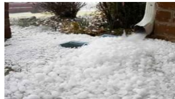
with hail storm damage
